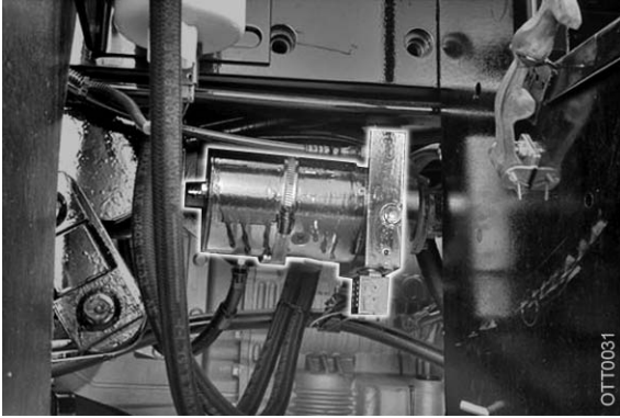
Electric Pump Motor — Cab Tilt System
